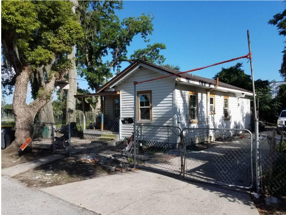
Existing building at 2101 Jerusalem Street
